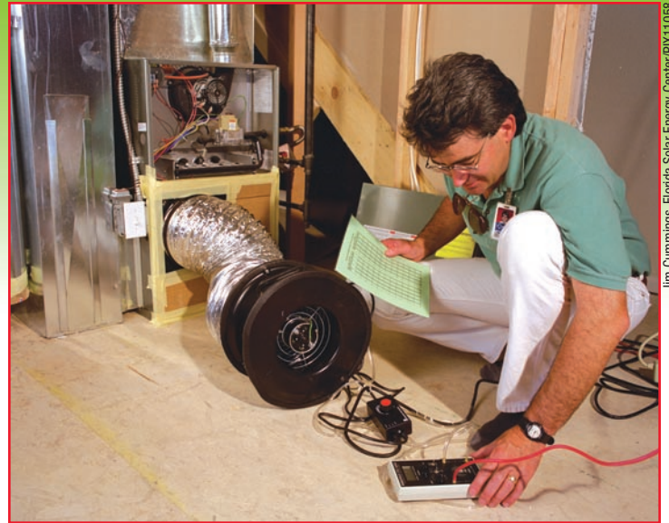
In this photo, a Building America staff member performs a duct blaster test to measure the impact of duct leakage on whole-house performance.
